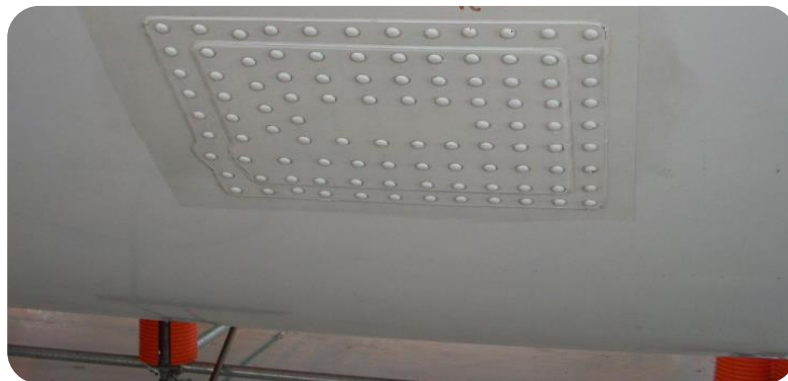
Figure 6. Riveted patch repair on Boeing fuselage.
