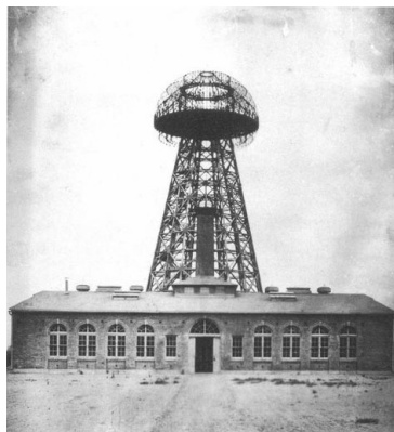
Figure 4.1: Teslas Wardencliff Tower (1904)
