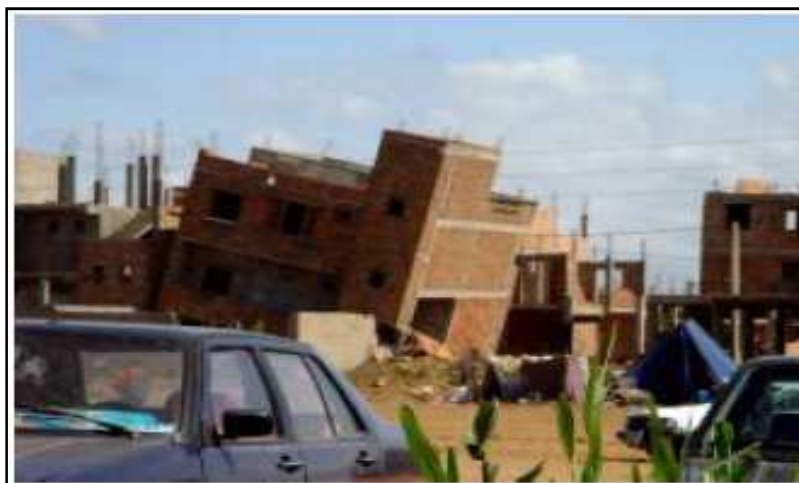
Photo B-I-8: Construction individuelle [8]
